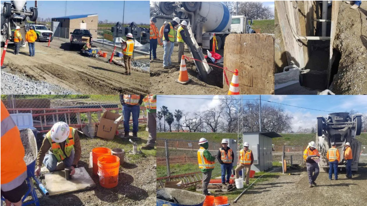
Reach B: Pumping Plant No. 3 Relief Well Controlled Low Strength Material backfill
