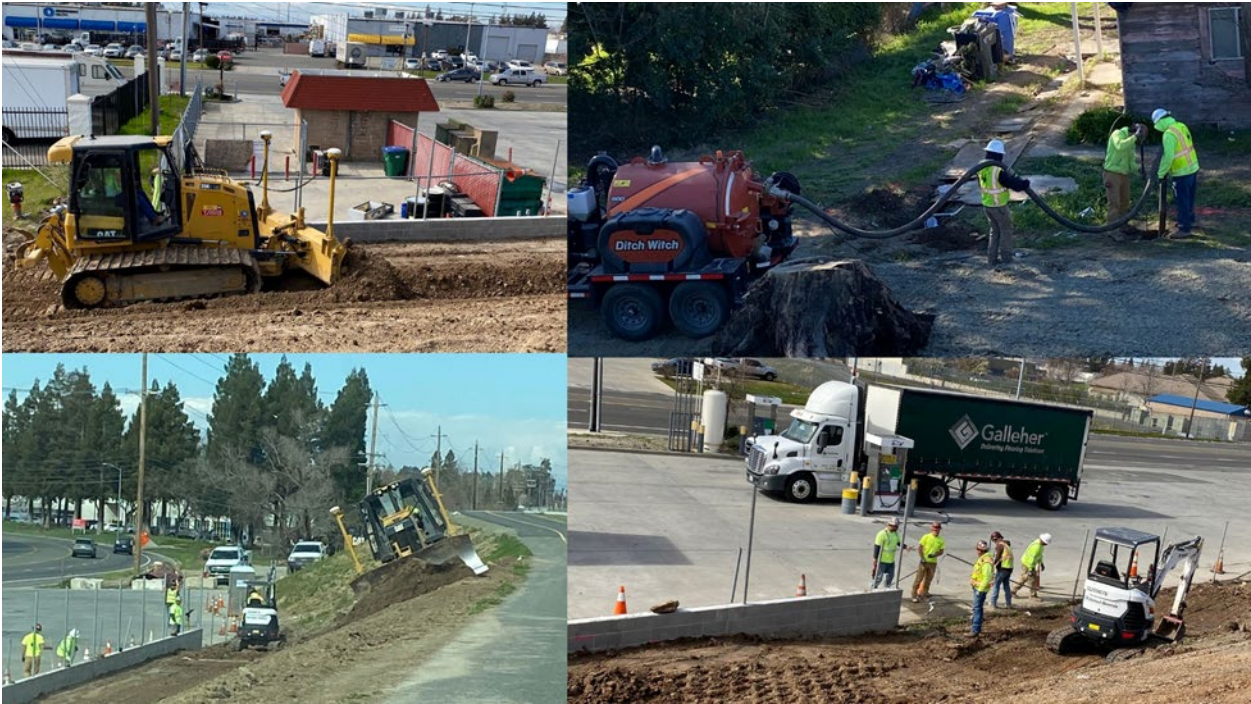
Reach H: Levee improvements and Seepage Berm construction
